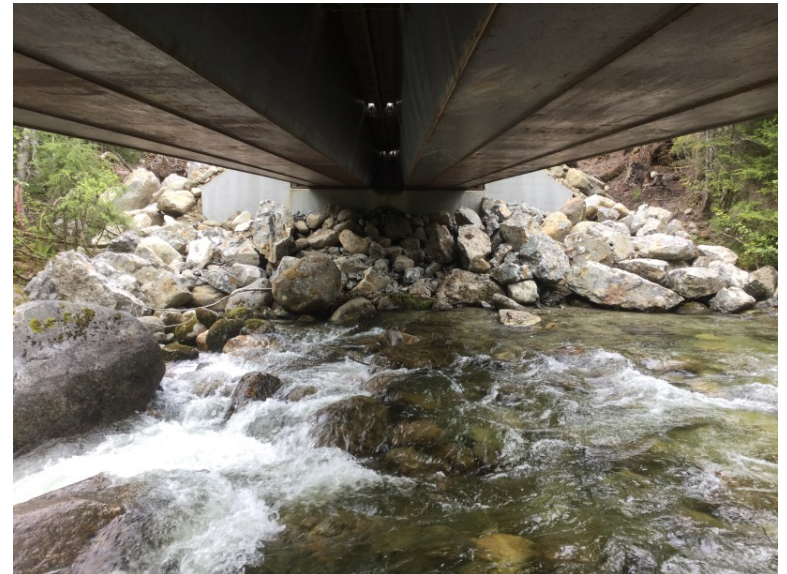
Right Bank Abutment when facing downstream
