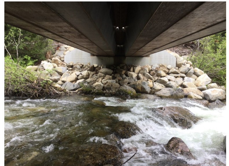
Left Bank Abutment when facing downstream
