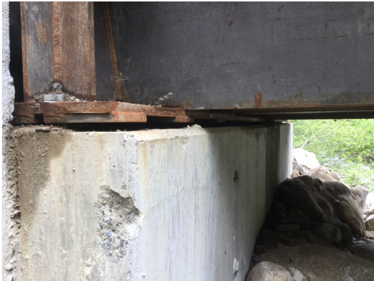
Upstream left bank shims
